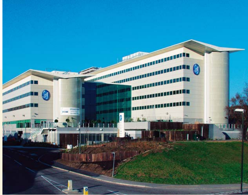
Above : Arora International Hotel, Garwick / Crawley, UK Architect: Arora development Product : HunterDouglas® QuadroClad
